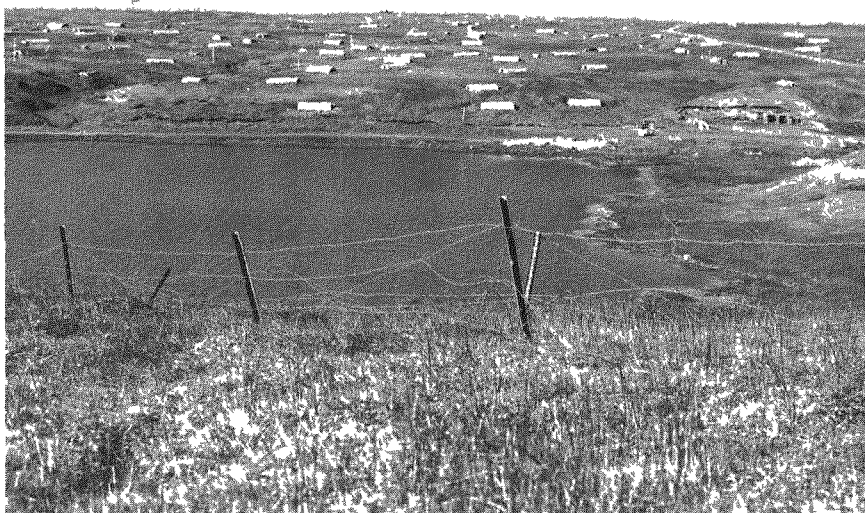
Fig. 9.5 Amchitka Island showing some of the buildings and roads remaining after the occupation by U. S. military forces.
